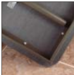
Tops are reinforced against breakage with a square corner steel frame.
